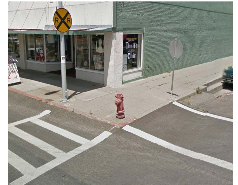
Examples of missing curb ramps or curb ramps that are not per code along Walker Street. Examples here are at 5 th and Walker Street and the alley in between 5 th and 4 th Street.
