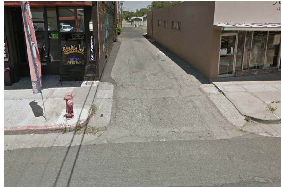
Examples of missing curb ramps or curb ramps that are not per code along Walker Street. Examples here are at 5 th and Walker Street and the alley in between 5 th and 4 th Street.
