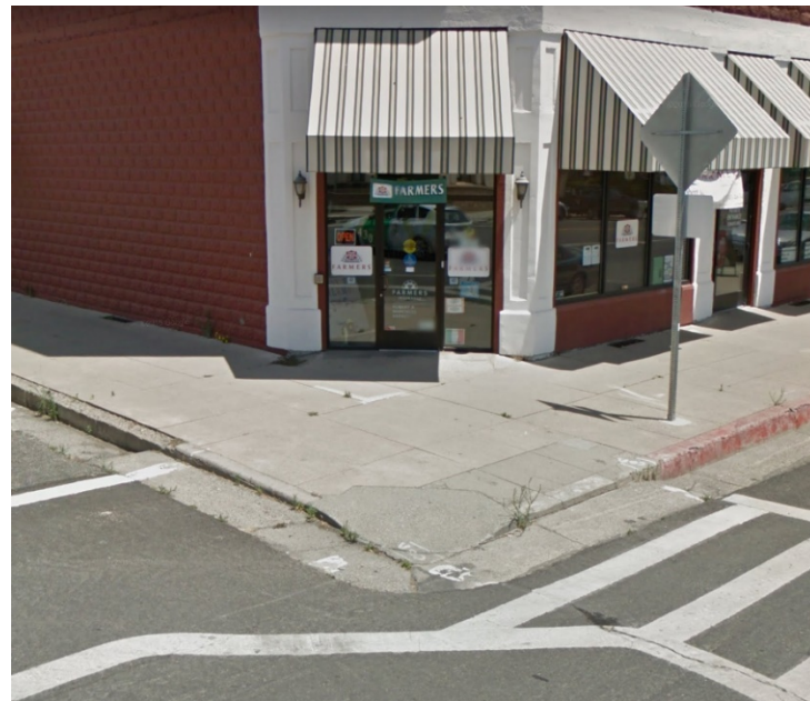
Examples of missing curb ramps or curb ramps that are not per code along Walker Street. Examples here are at 5 th and Walker Street and the alley in between 5 th and 4 th Street.
